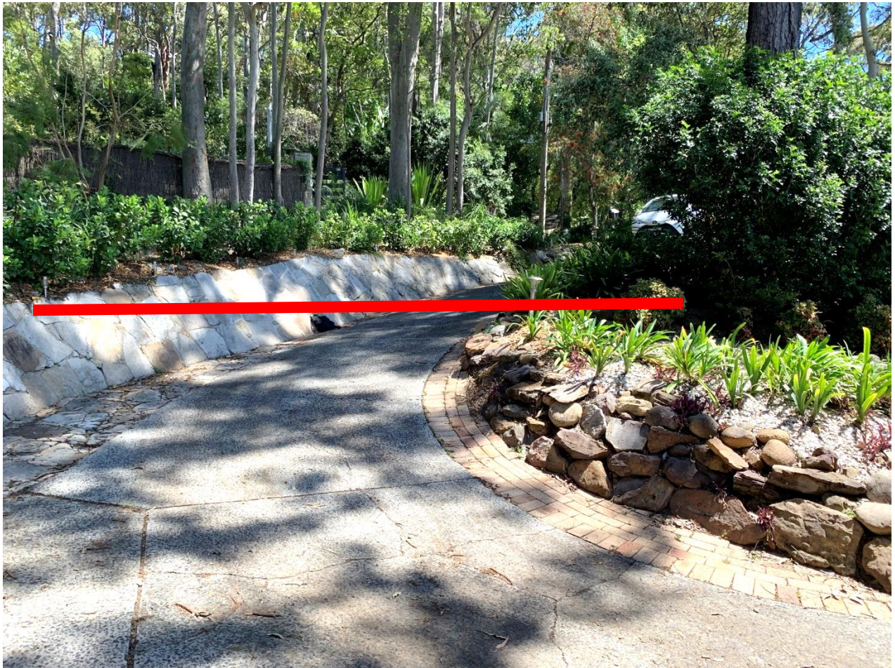
Figure 5: The carport and driveway level will be roughly at the red line. The remaining old concrete of the driveway will be removed and made as an area of new garden. New steps and garden paths are designed to be elevated above existing ground levels and require no excavation.
