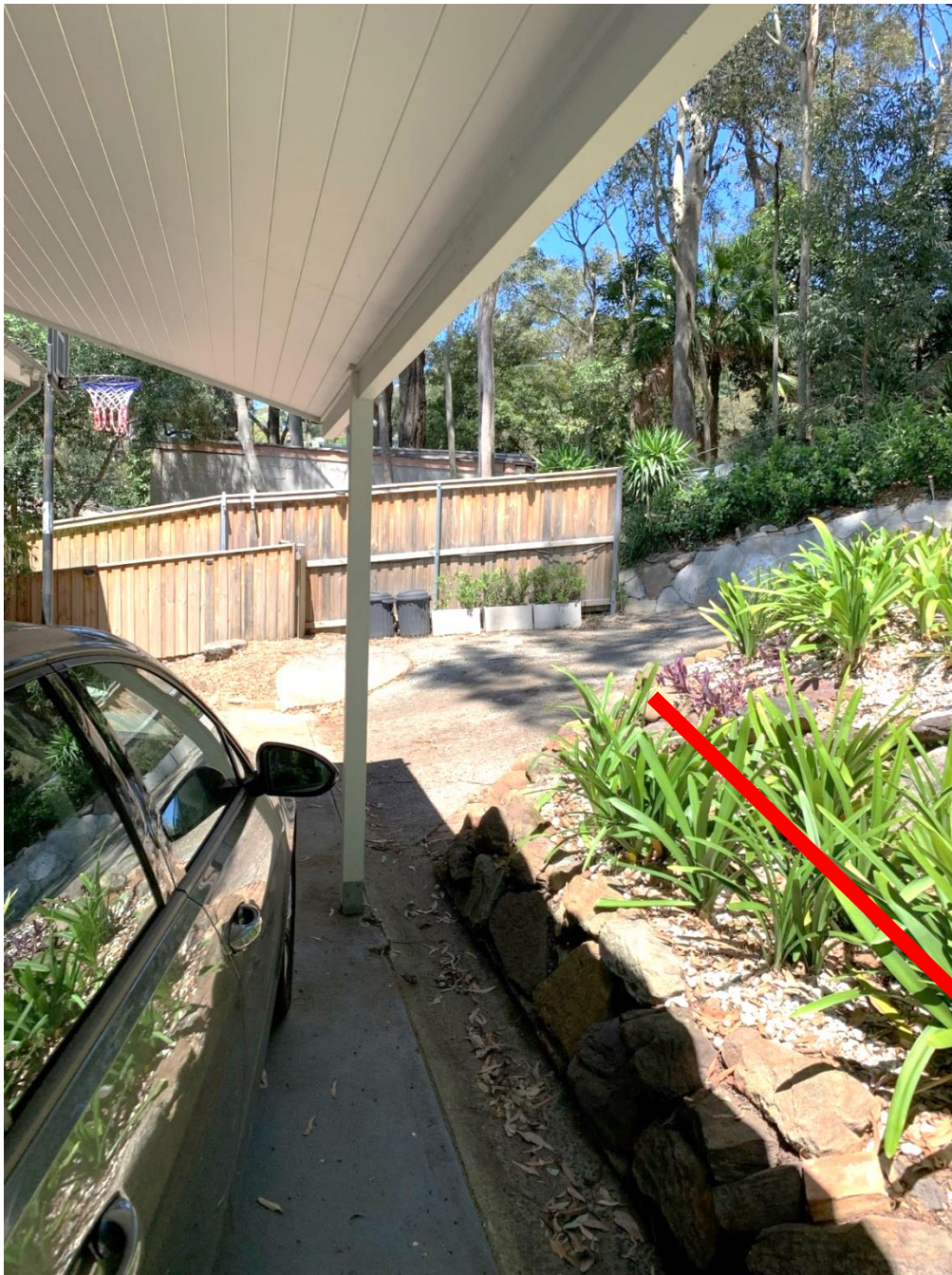
Figure 4: The old carport is to be removed, and the old stone retaining wall at the toe of the bank is proposed to be removed and the bank cut back by one metre, roughly along the red line. This is 5 metres from the tree and downhill of the tree. Theoretically the tree will have most of its tension roots located uphill of the stem, so it is anticipated that this excavation will not have a detrimental impact on the trees' stability. However, care should still be taken to hand excavate the line of the proposed cut, as it is within the Tree Protection Zone. If a significant number of large diameter roots are encountered then an alternative design may have to be considered to retain the tree safely.
