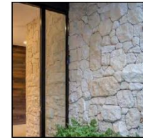
5 - STONE FEATURE CLADDING: FINISH TBC BY CLIENT
