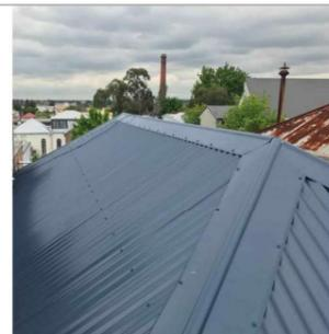
ENSURE ALL NEW ROOFING MATERIALS, SYSTEMS OR ACCESSORIES SHALL BE NON-COMBUSTIBLE, AND SEALED IN ACCORDANCE WITH AS3959:2018 CLAUSE 3.6
