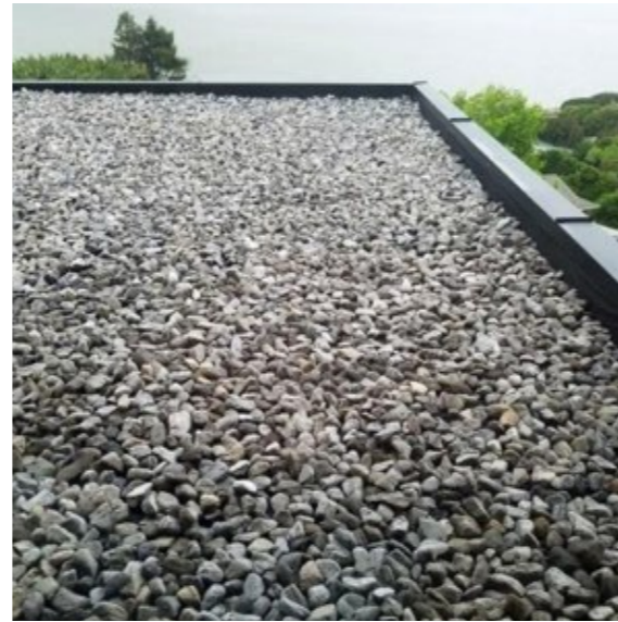
RF-01 - MEMBRANE / BALLASTED ROOF
