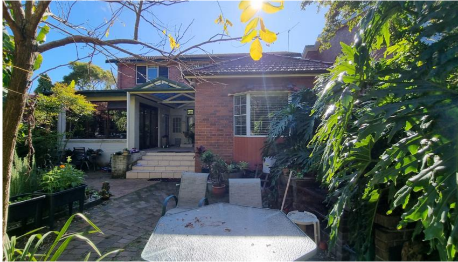
Photograph-5: View of rear side of the main building at 54 Brighton Street. View looking north from the rear yard.
