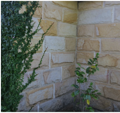
CL-03 CLADDING 03 SYDNEY SANDSTONE CLADDING
