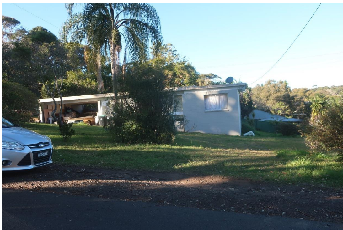
Figure 4.24 View of residential building on Lot 3 along The Avenue, facing south. AMAC Group IMG_7395 (21/06/2023).
