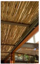
EXAMPLE: TIMBER BATTEN TO PERGOLA
