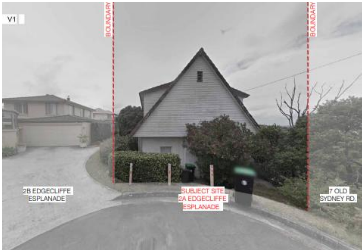
Figure 3: Subject property as viewed from Edgecliffe Esplanade with the public walkway located to the left of the dwelling house
