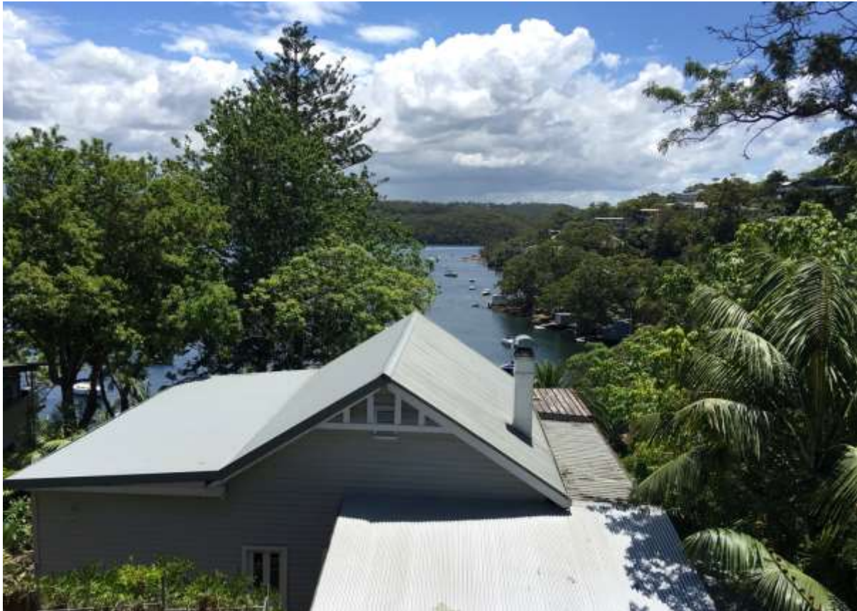
Devastating View Loss from Highly Used Room: Lower Level
