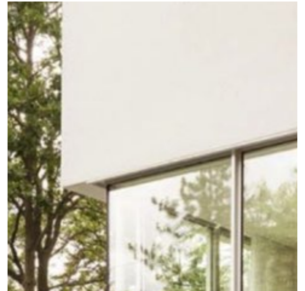
WD-01 - ALUMINIUM WINDOWS RB-01 - RENDERED CONCRETE BLOCK
