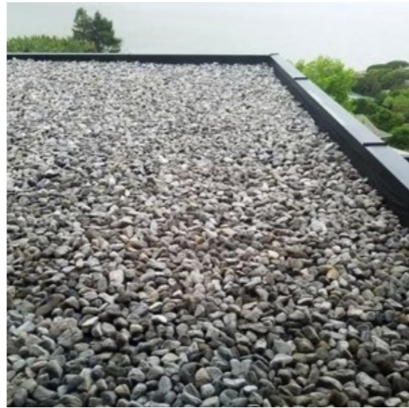
RF-01 - MEMBRANE / BALLASTED ROOF
