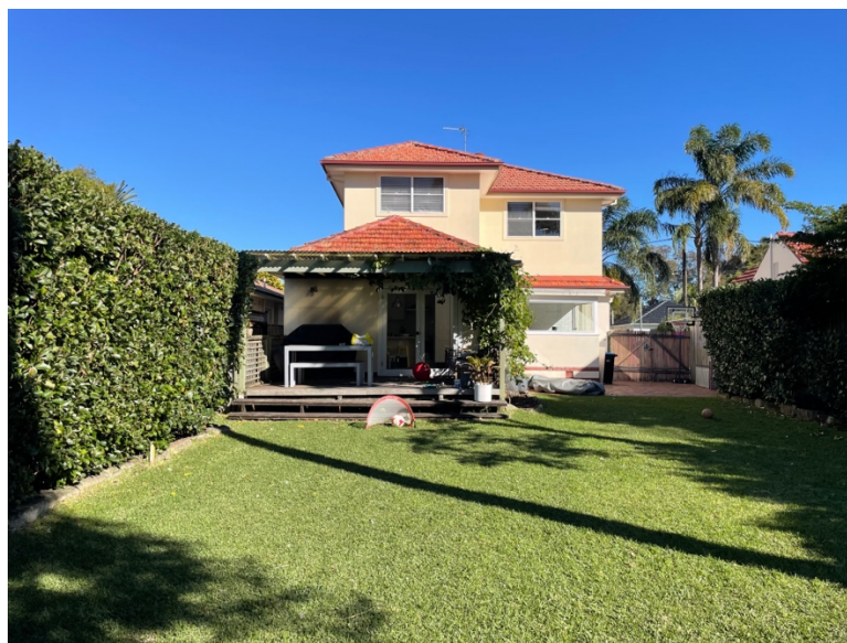
Rear View of Existing Dwelling
