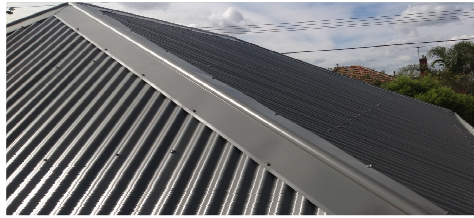
BLUESCOPE STEEL COLOURBOND CUSTOMORB ROOF SHEETING AND CAPPINGS. COLOUR TO COMPLY WITH BCA CLASSIFICATION OF DARK (SOLAR ABSORPTANCE 0.475 - 0.70)
