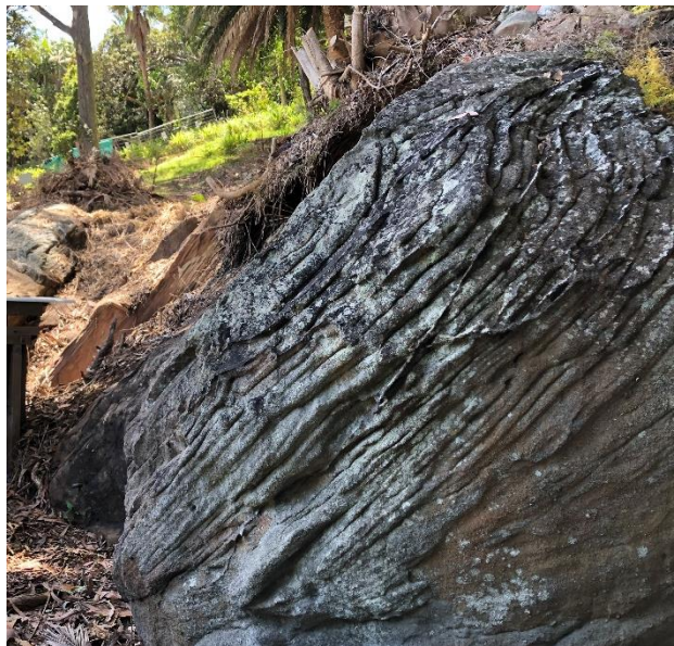
Photograph-4: Sandstone boulder and wash out under roots of palm tree, looking north east
