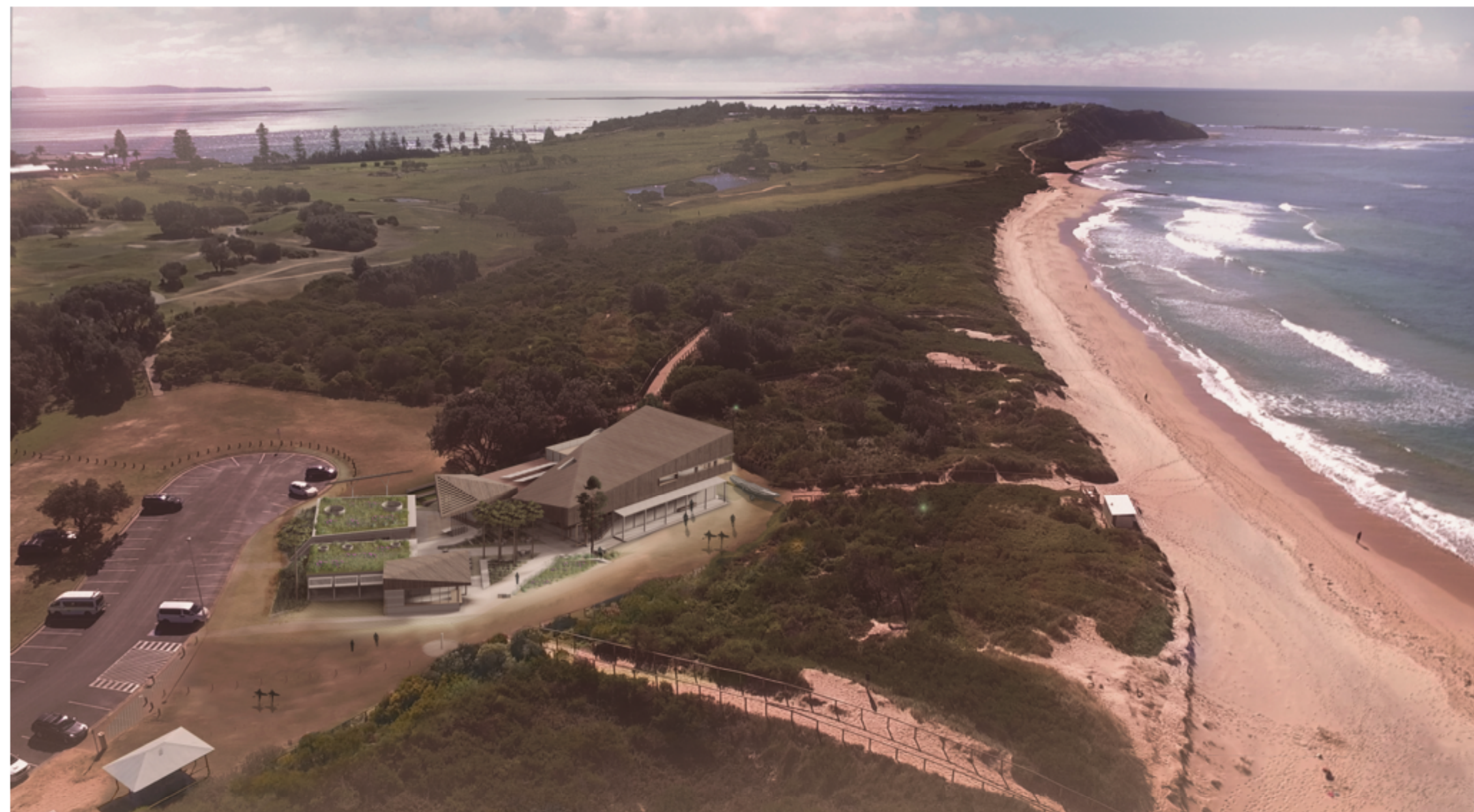
Montage 1 - Aerial view
