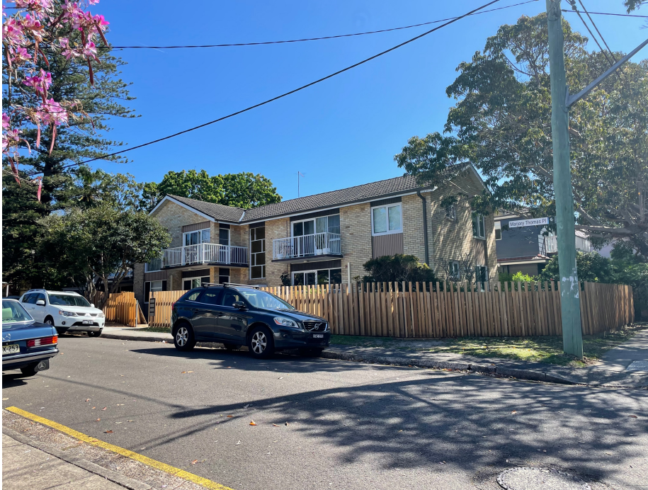
Figure 2: Balgowlah Road frontage
