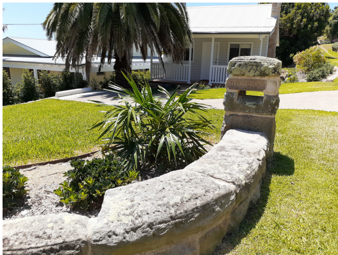
This original wall is 300mm high
