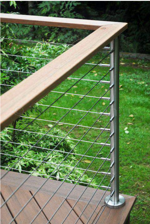
WIRE BALUSTRADE WITH TIMBER HANDRAIL
