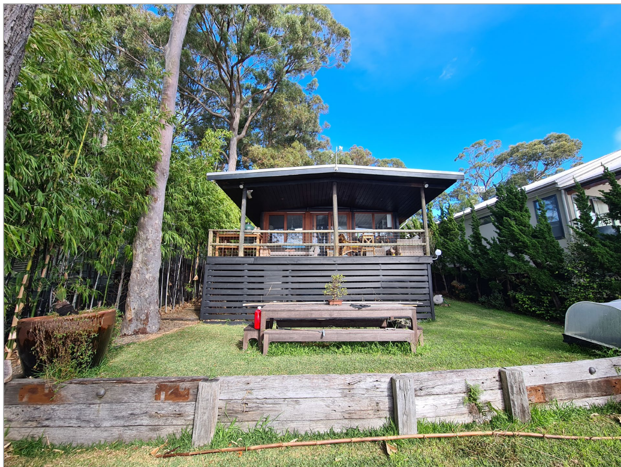
Photograph 1: Northern side of existing dwelling
