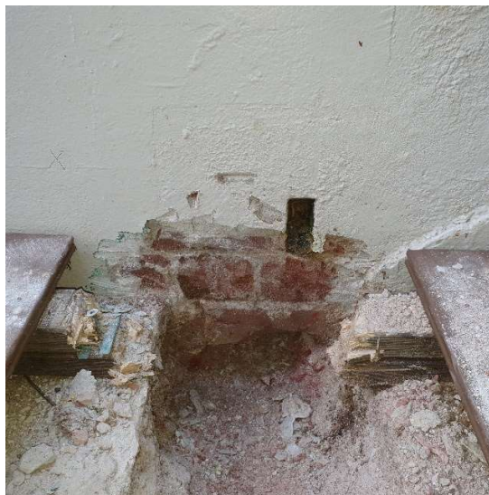
Photograph-12: TP1 excavation. View looking down west.
