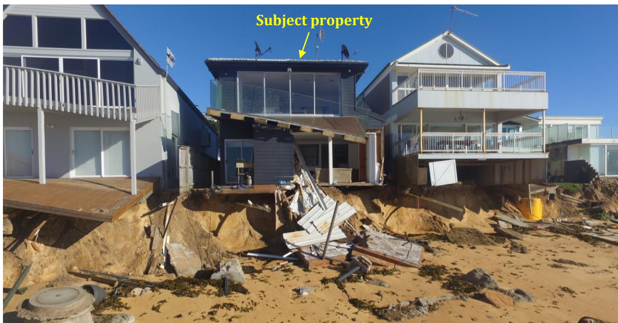
Figure 2: View of subject property on 10 June 2016, facing approximately west, with the leaning first storey deck subsequently removed (photograph supplied by UNSW Water Research Laboratory)
