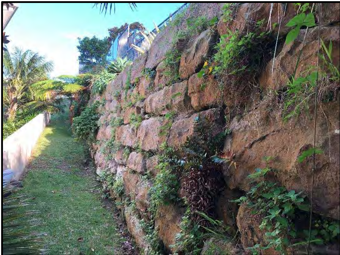
Photo 6 – View along southern boundary of No. 41, looking west.
