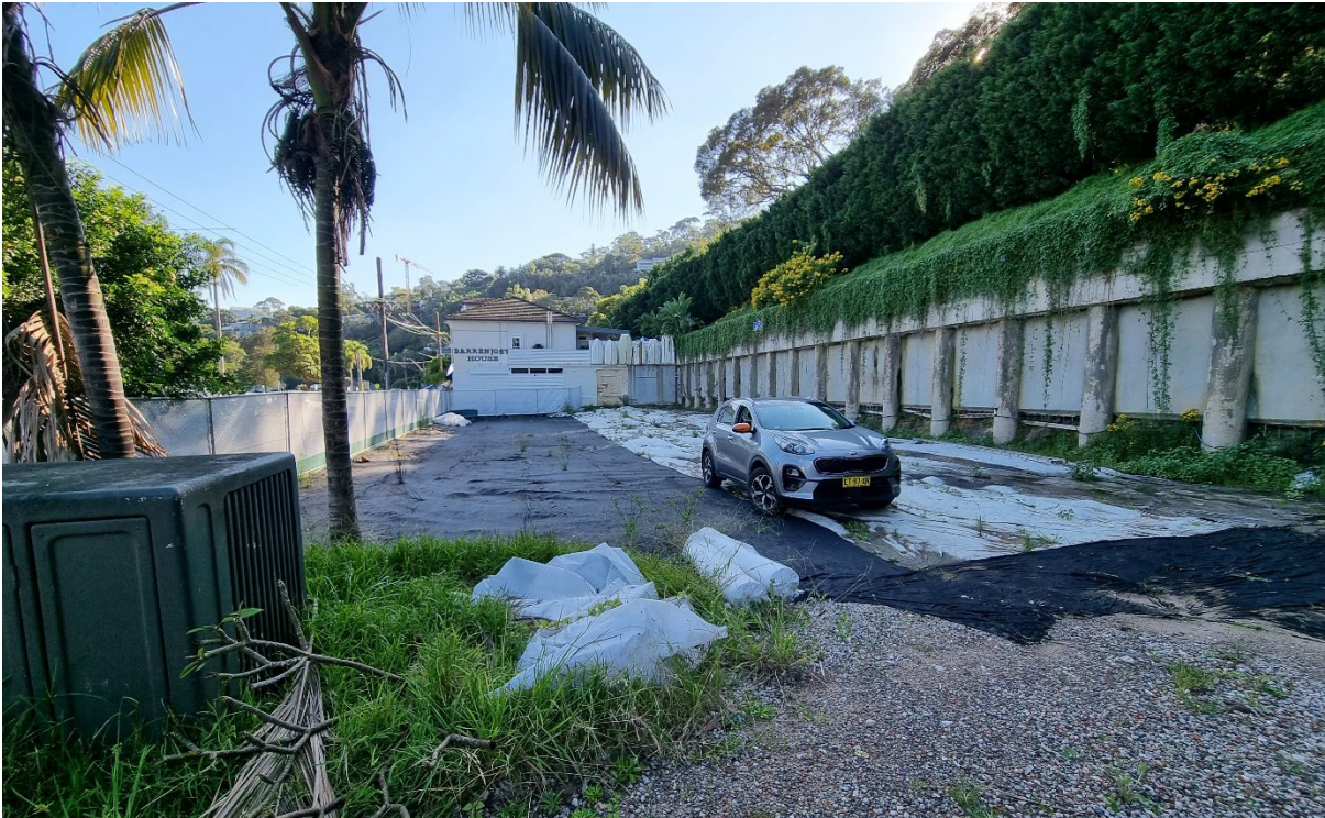
Plate 1. Site layout, facing north. Ground covering and scarp with soldier pile wall evident, as well as electricity kiosk.
