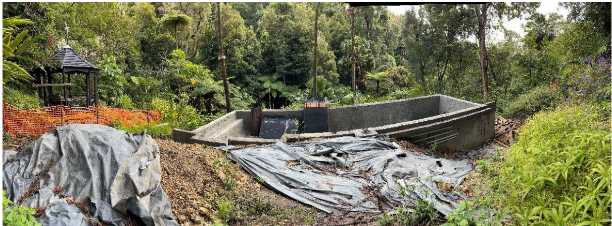
PHOTOGRAPH 5 - THE CONSTRUCTION OF THE PROPOSED SWIMMING POOL (VIEW TO NORTH)
