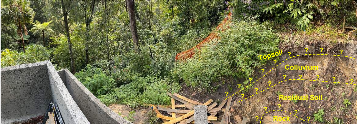
PHOTOGRAPH 6 - EXPOSED GROUND CONDITIONS AT THE LOCATION OF THE ART STUDIO (VIEW TO NORTHEAST)
