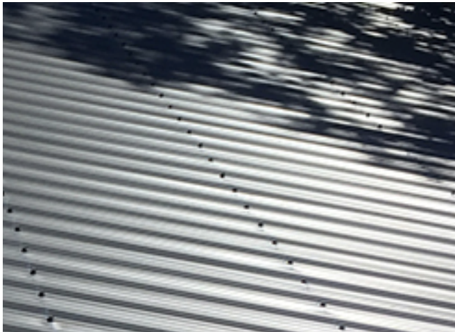
CB - COLORBOND 'SURFMIST' ROOF SHEETING OR SIMILAR
