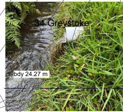
Photo: hose water runs into creek below house
