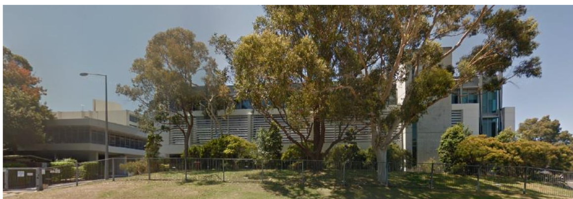
Figure 4 The existing building to the south of the retained former Roche office building. Source Google Streetview.
