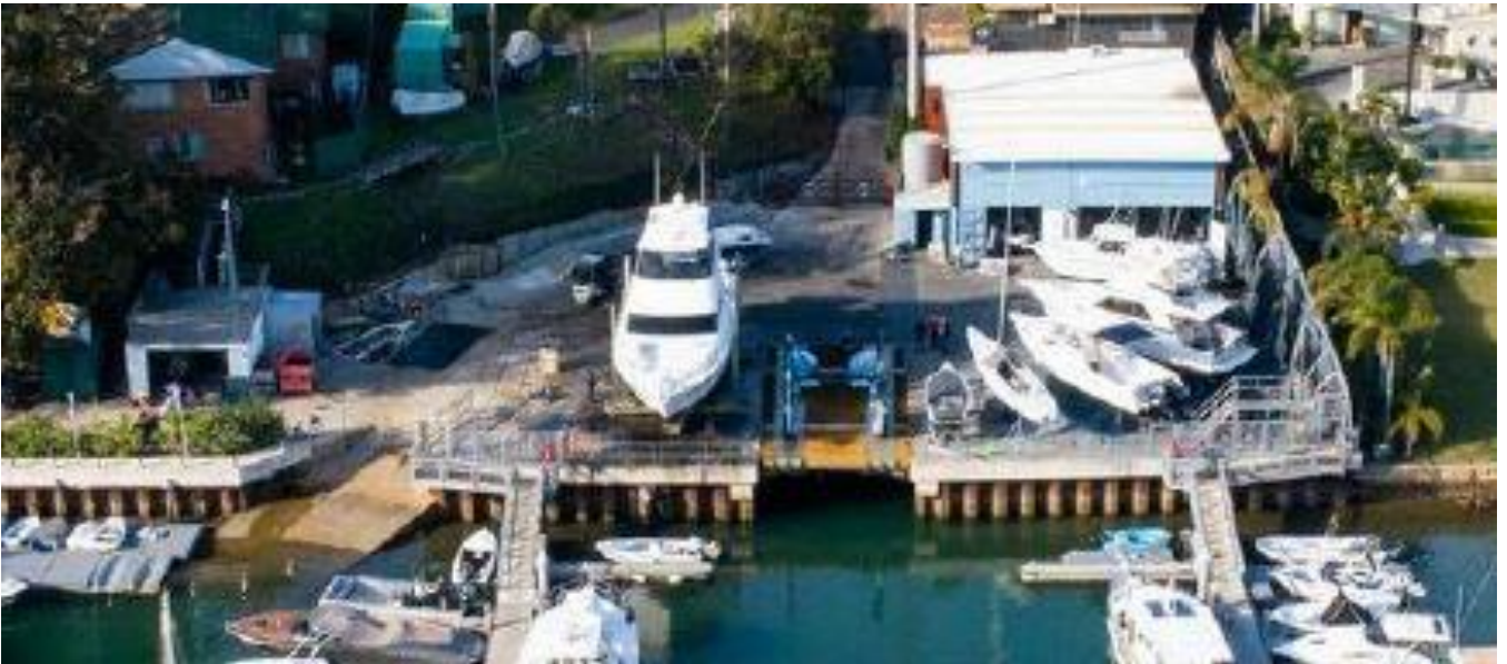
Figure 7 Existing Sirsi Marina condition ramps, pontoons and vertical slipway.
