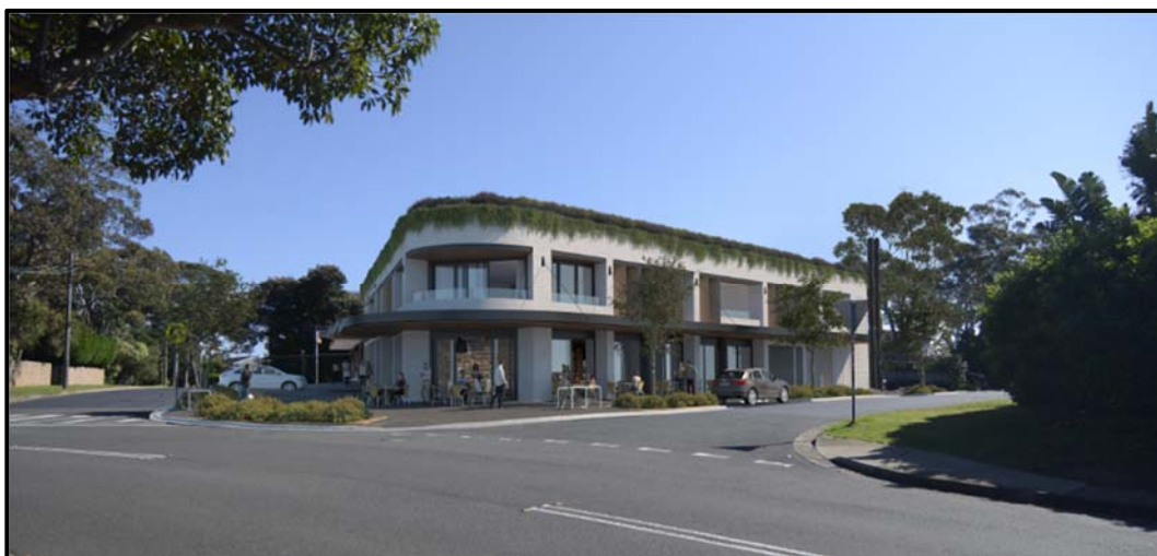
Figure 4: 3D view of proposed looking from Plateau Road, with Bilkurra Avenue on right (Source: Benson McCormack Architecture, Project No. 2012A)
