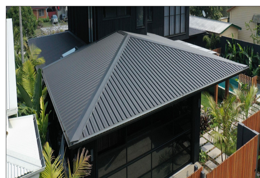
3. COLORBOND MONUMENT METAL ROOF
