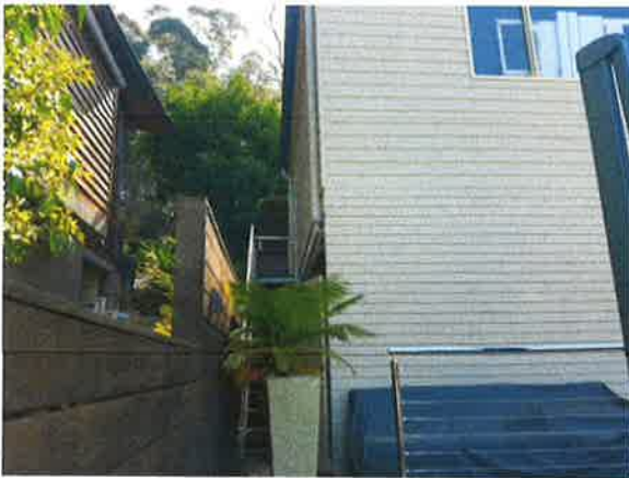
Existing garage, looking N along boundary
