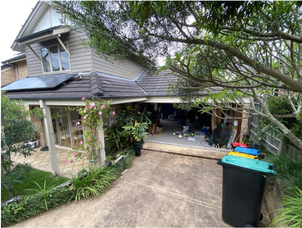
Figure 6. The existing driveway, garage and dwelling facade, looking east
