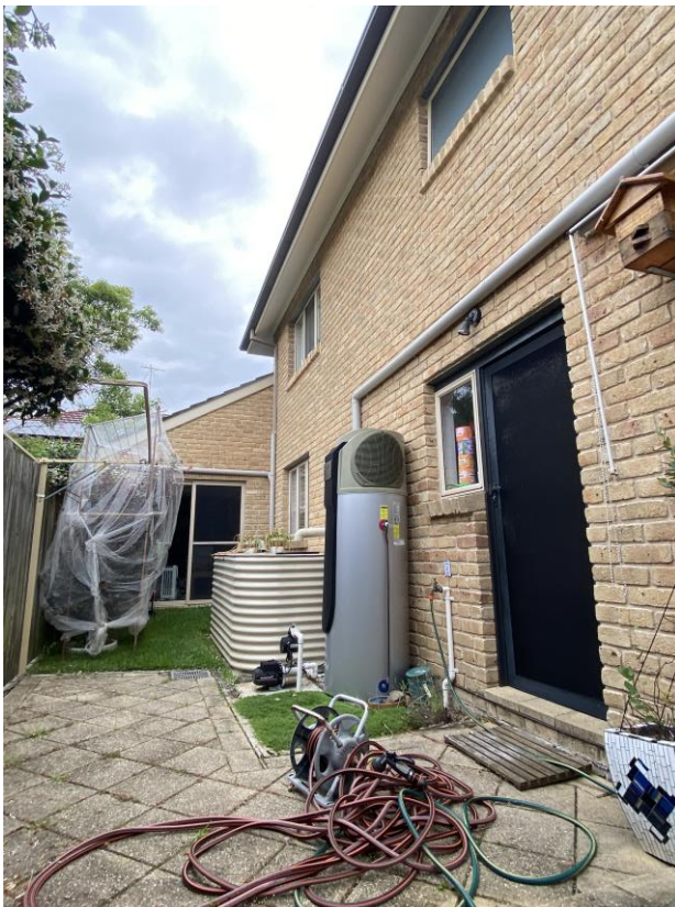
Figure 9. The rear elevation of the existing dwelling, looking south
