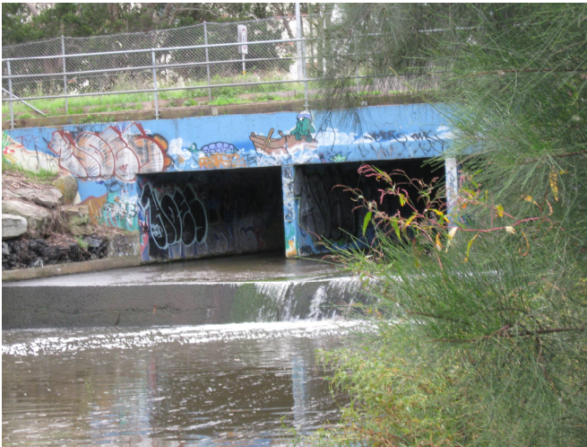
Plate 2 Condamine Street Culverts
