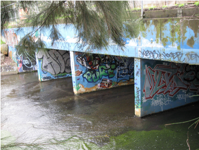
Plate 1 Condamine Street Culverts
