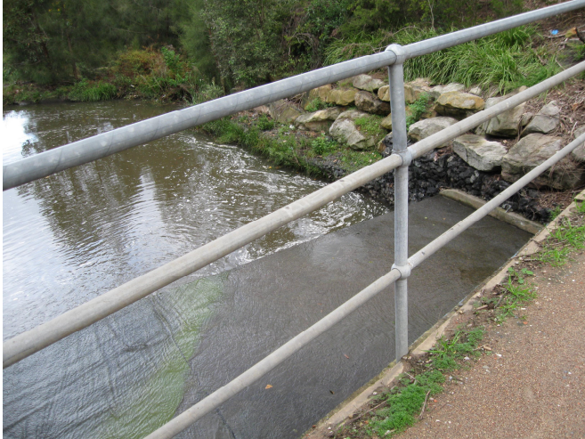
Plate 4 Downstream Apron /GPT Pool
