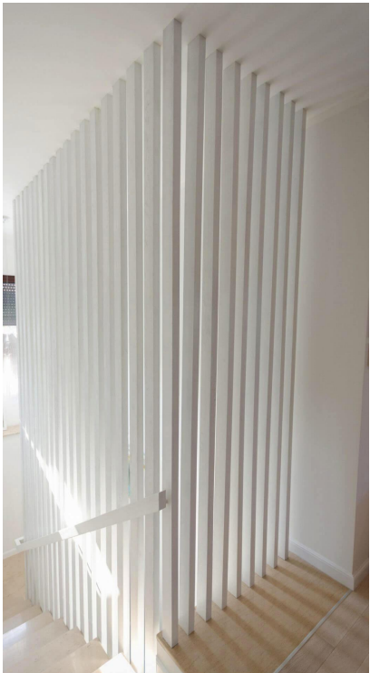
3. Vertical Timber Battens
