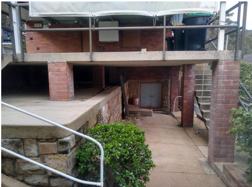
Photo 2: View underneath secondary residence
