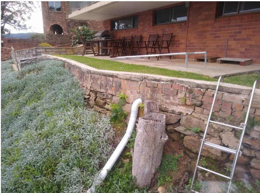
Photo 5: View looking at main residence and retaining wall below (view north)
