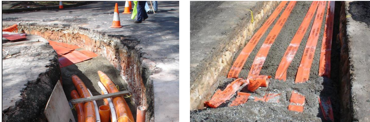
Figure 10 – Thermally stable bedding during installation works
