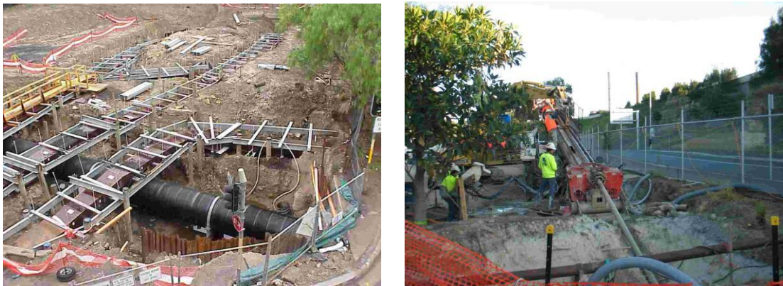
Figure 5 – Work below surface level
