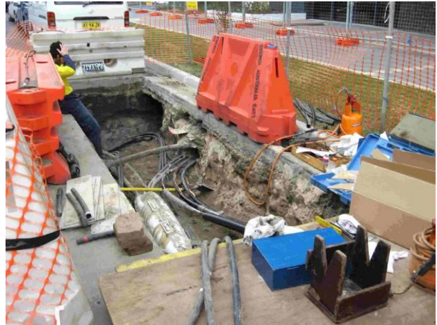
Figure 2 - Photo of typical joint bay
