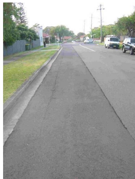
Figure 12 – Permanent reinstatement
