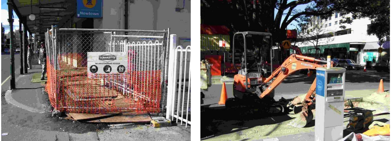
Figure 9 – Excavation and removal of sub-surface material
