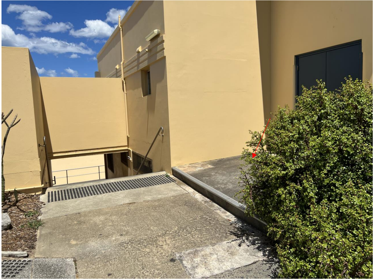
Figure 2: View of location of proposed works (at arrow), facing SSE, on 21 November 2022
