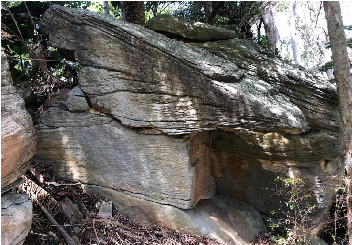
Photograph-7: Two detached units bearing onto a mostly buried sandstone boulder, looking south
