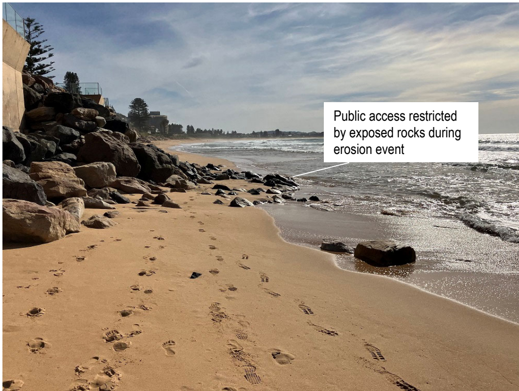
Figure 2-6 View along Collaroy Narrabeen Beach showing existing historic rock revetment at Wetherill Street exposed following erosion event and extending onto beach
