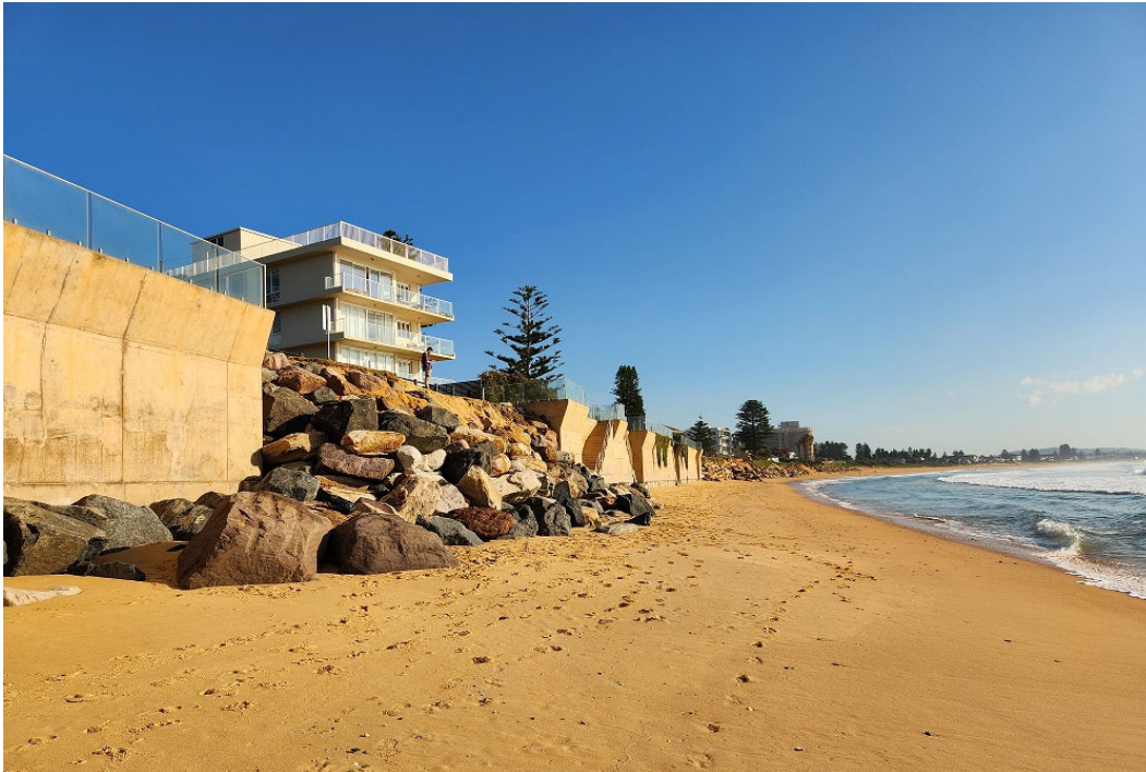
Figure 2-7 Upgraded private coastal protection works at 1168 and 1172 Pittwater Road
