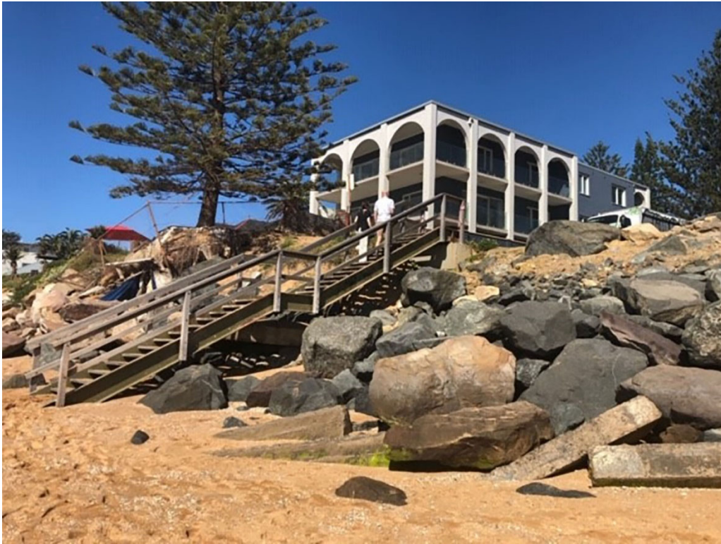
Figure 2-4 1168 Pittwater Road with rock revetment and now removed access stairs in the foreground (2020), taken prior to commencement of upgraded private coastal protection works
