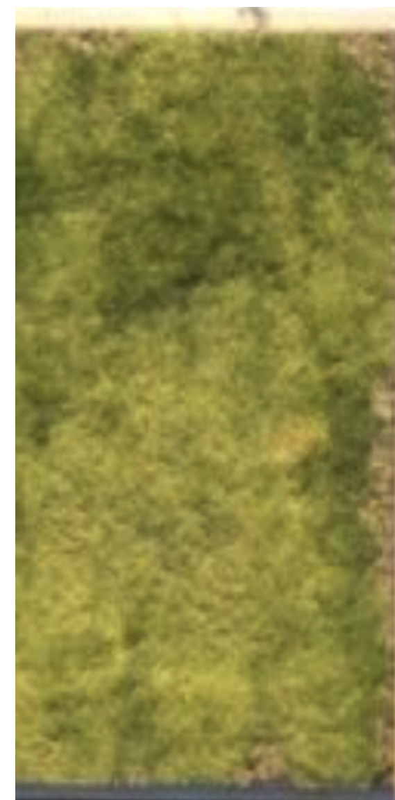
EXTENSIVE GREEN ROOF
