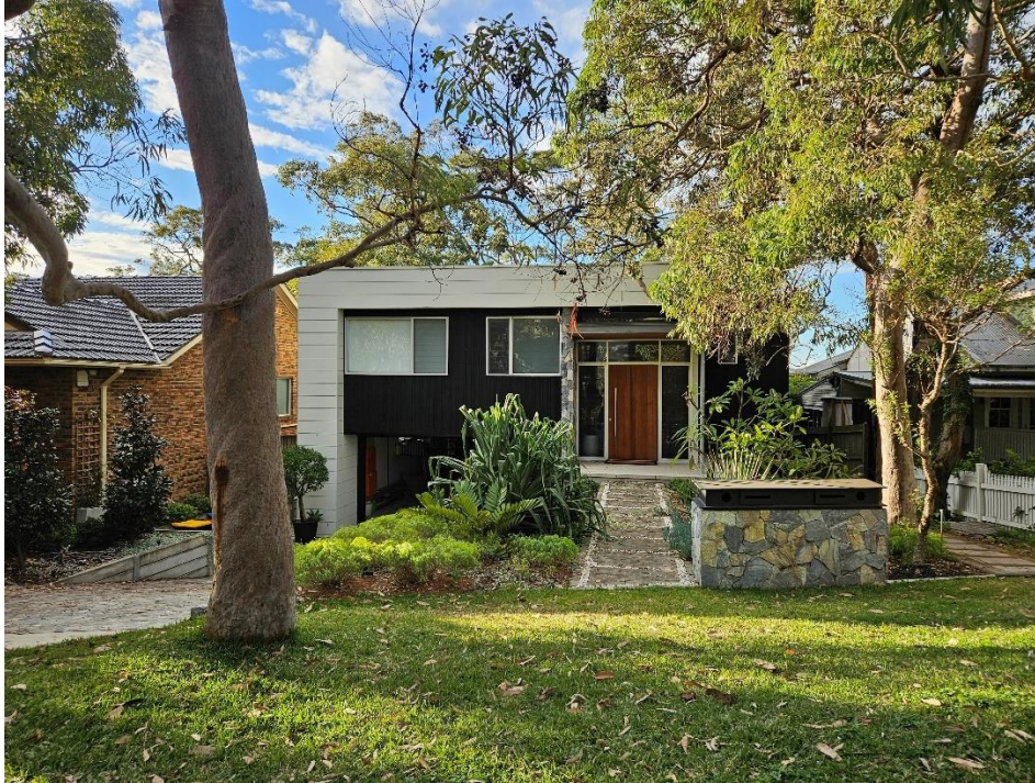
Existing Property no. 74 Queens Parade East Newport to the West of the subject site
