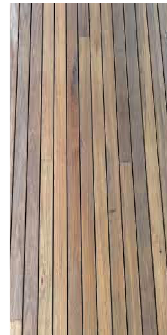
HARDWOOD TIMBER DECKING STAIRS
