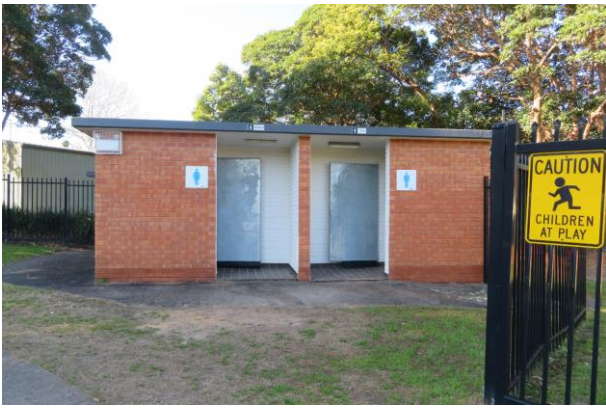
Figure 31 – View of the toilet Block in the north west corner of the Oval site.
