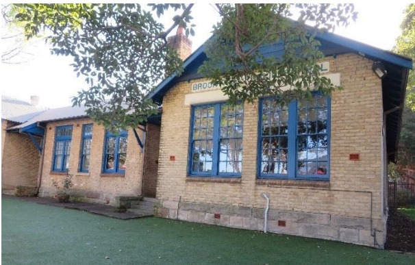
Figure 13 – Detail of heritage item, Brookvale Public School
