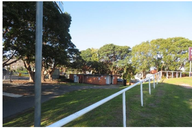
Figure 32 – View east of the toilet block in the north west corner of the Oval.
