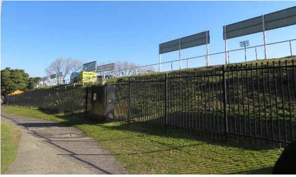
Figure 17 – View south-west showing the berm which constitutes the eastern spectator stand.
