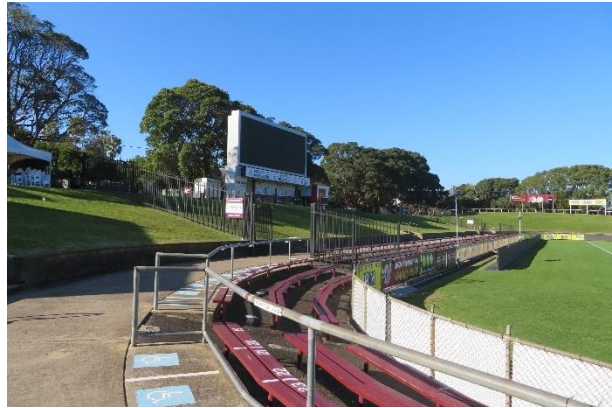
Figure 36 – Detail of bar on the northern Oval boundary topped by a screen.
