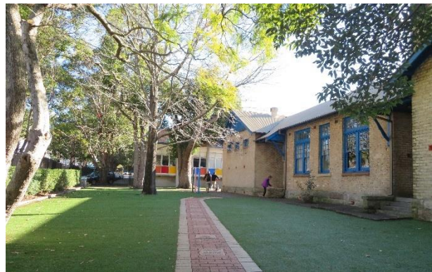
Figure 14 – View west across Brookvale Public School
