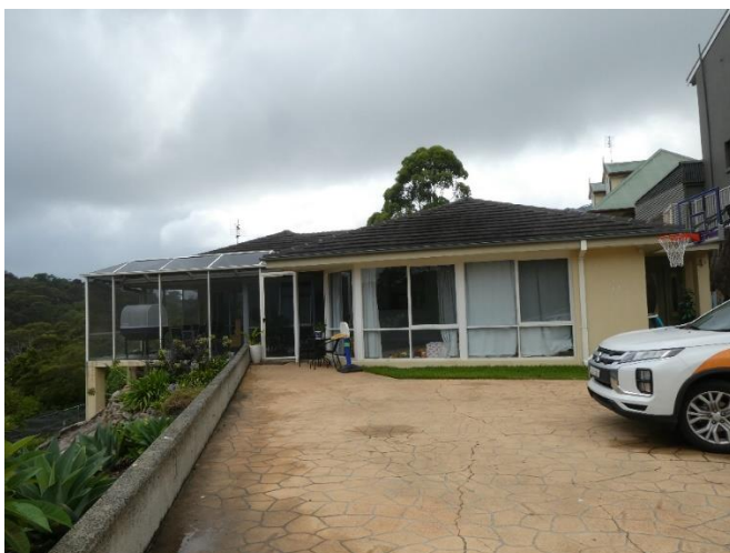
Image 1: NORTH VIEW OF THE EXISTING DWELLING – NEW DECK EXTENSION/PATIO AREA WITH NEW ENTRY EXTENSION AND LOCATION. PORTION OF PAVING TO BE REMOVED TO REINSTATE LANDSCAPING.
