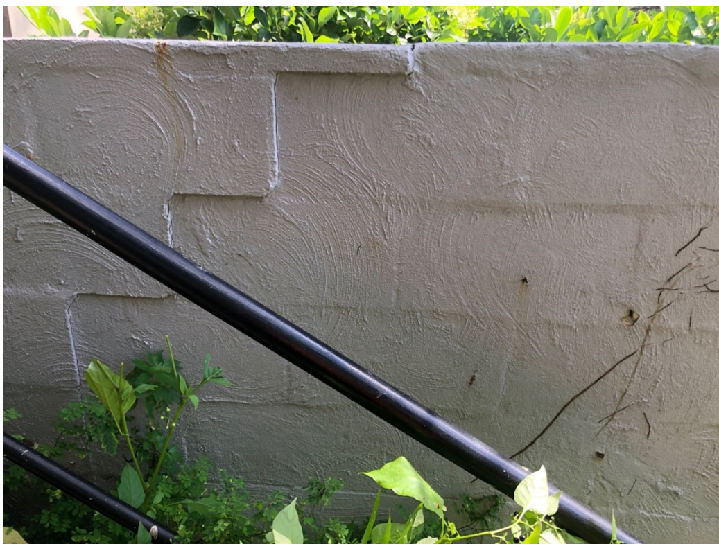
Figure 1: Crack in Northern Boundary Wall
