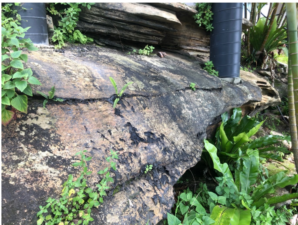
Figure 6: Pier on undercut rock shelf viewed to the north
