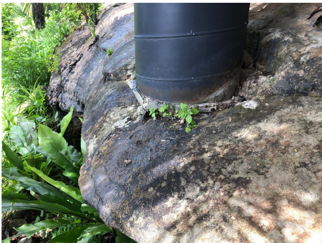
Figure 5: Pier founded above rock overhang
