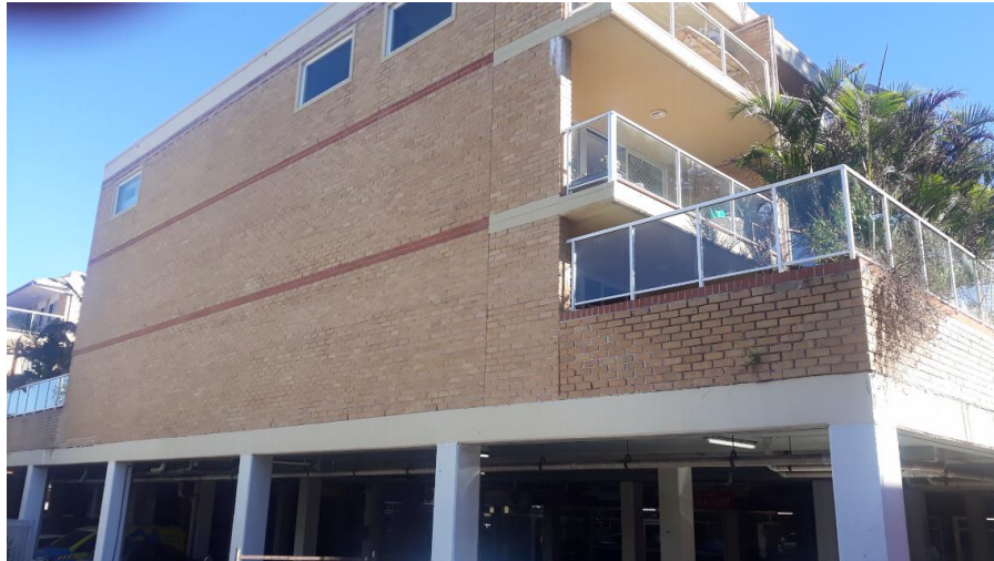
Photo 1 View of 1-5 Collaroy Street Adjoining the Rear Boundary of the Development Site
