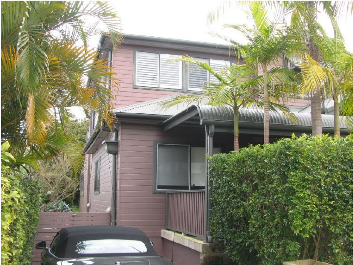
Figure 2: Street view of subject site
