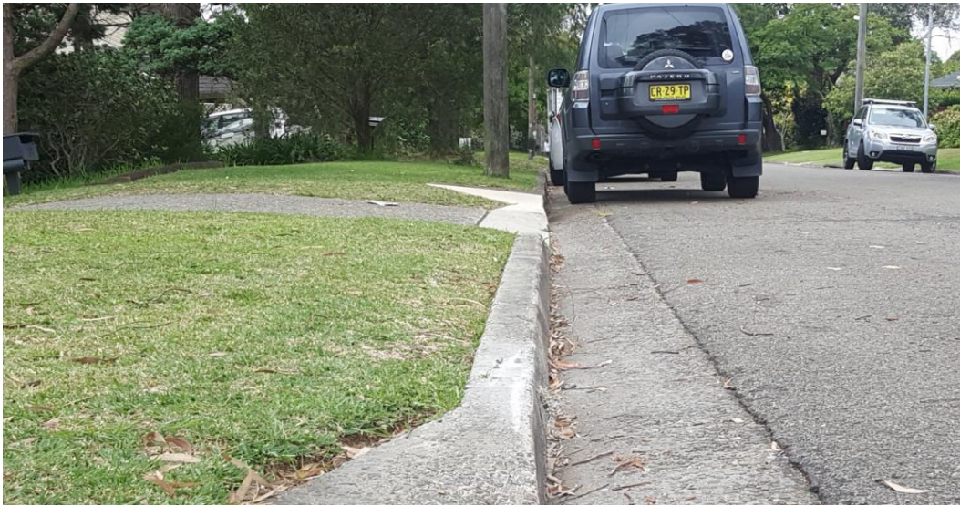
Figure 2. Grass crest present if overland flow toppled the kerb (pit located behind Mitsubishi).
