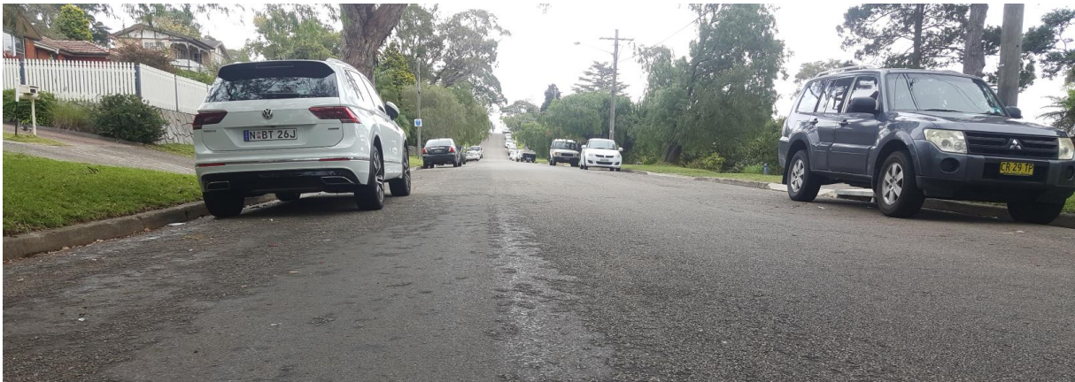
Figure 4. Existing pit's (RHS under Mitsubishi) overland flow route if pit surcharged (12 Dareen Street- photo looking upstream)
