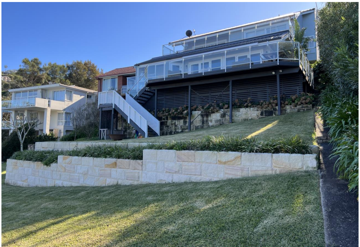
Figure 4: View of seaward portion of subject property on 25 June 2022, facing NNW
