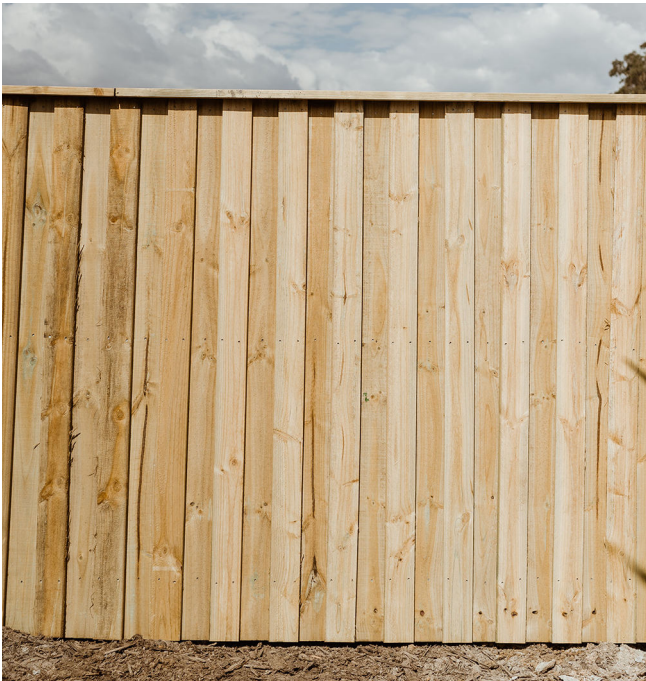
Lapped & Capped Fence Location: South Boundary
